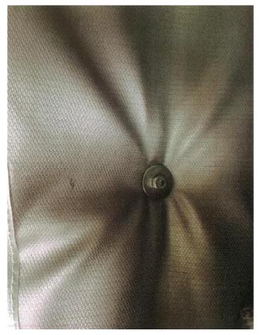
C. On the inside of door frame it may be necessary to remove a small piece of insulation to get the washer and lock nut on the bolt.
